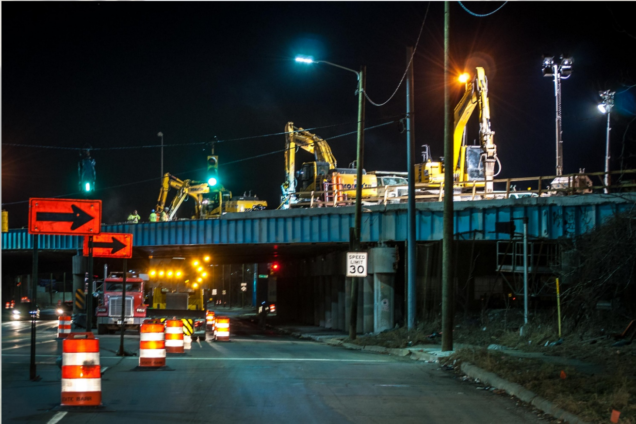
SB I-75 Fort Street Bridge Demolition Continues
