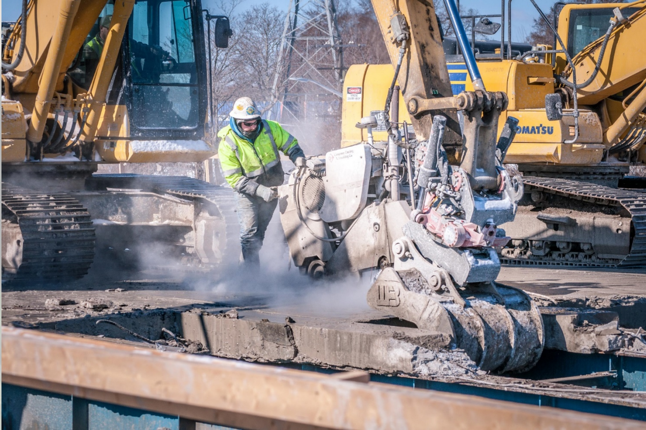
SB I-75 Fort Street Sawing and Slabbing Deck Demolition
