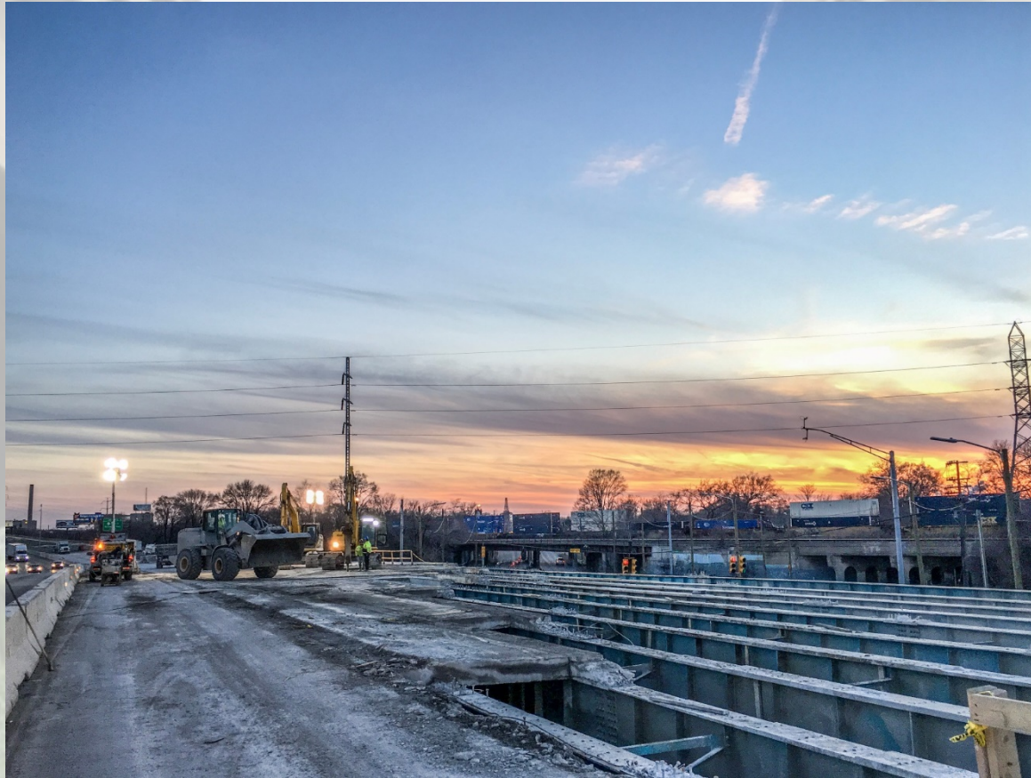
SB I-75 Fort Street Bridge Demolition Continues
