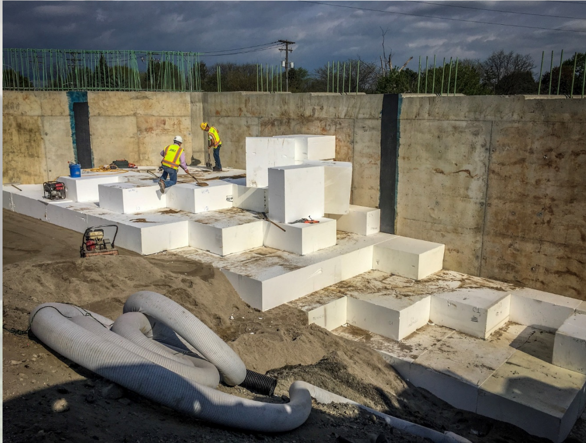
SB I-75 South of Goddard Installing Lightweight Fill
