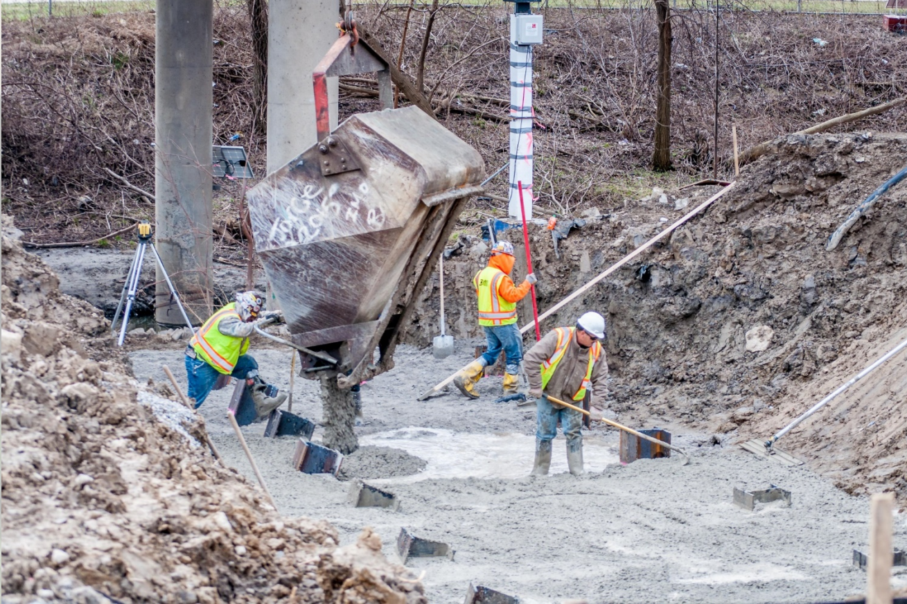
SB I-75 At Sexton-Kilfoil Drain Pouring Sub-footing for South Abutment
