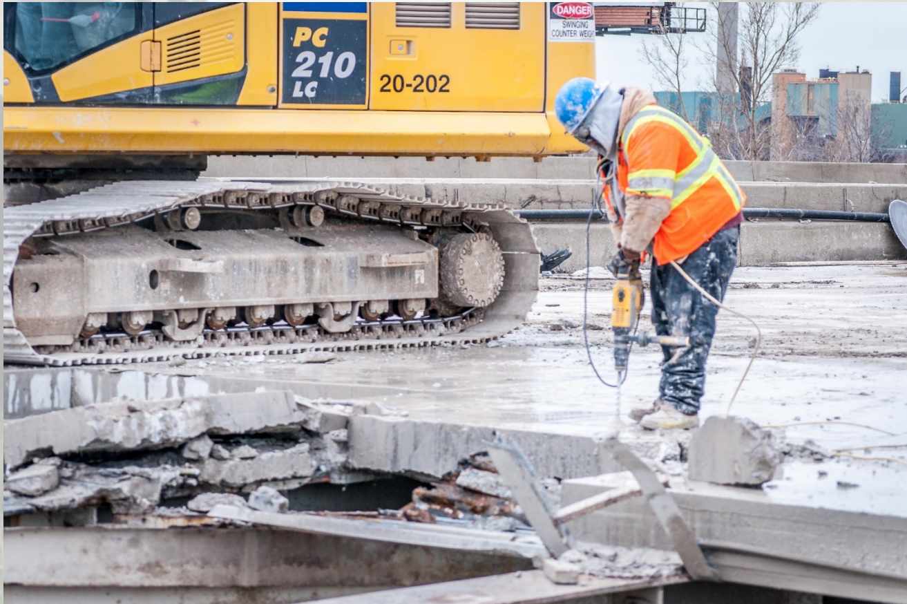
SB I-75 Rouge River Bridge Demolition Continues
