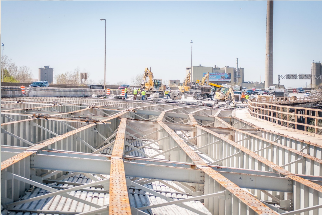
SB I-75 Rouge River Bridge Continuing Bridge Deck Removal
